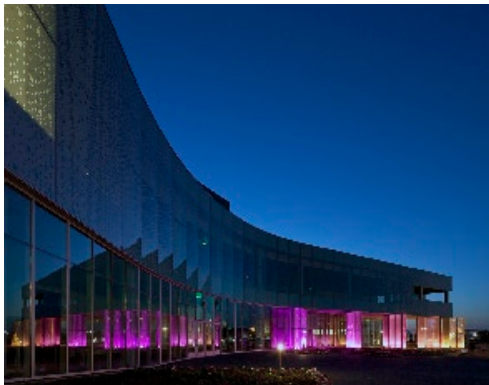
PANELITE™ IB-TC4 • Burnsville Performing Arts Center Design: Akeny Kell Architects • Photography: Jim Gallop
